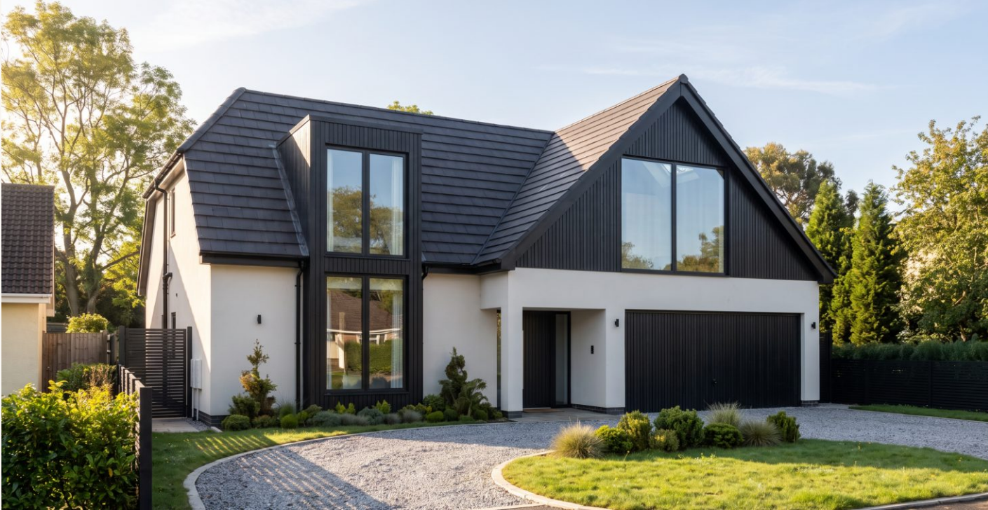
Front elevation, morning
